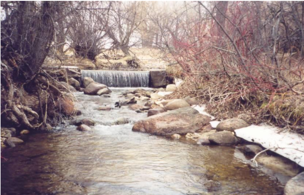
Figure 3-4. An example of an irrigation diversion structure used to route stream waters to irrigated hay lands.
